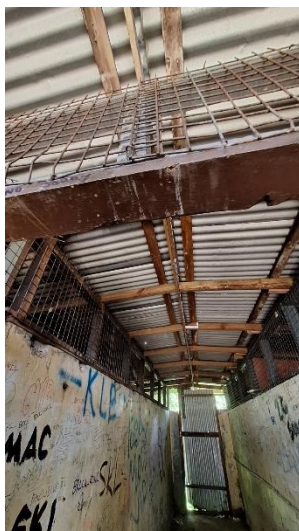
PHOTOGRAPH No. 5: EXPOSED TIMBER ROOF FRAME
