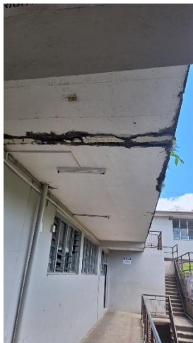
PHOTOGRAPH No. 3: WALKWAY AT TOP LEVEL WITH CONCRETE SPLIT AT ROOF BEAM
