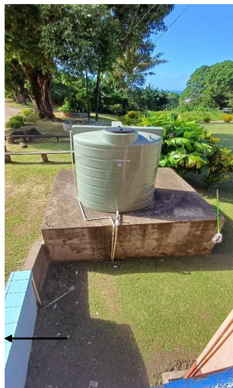
Figure 8: B1 WATER TANK WITH TAPS.
