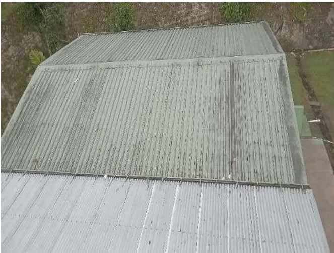
03. TRIMDEK ROOF CANTEEN, CORRUGATED ROOF WASH BAY.
