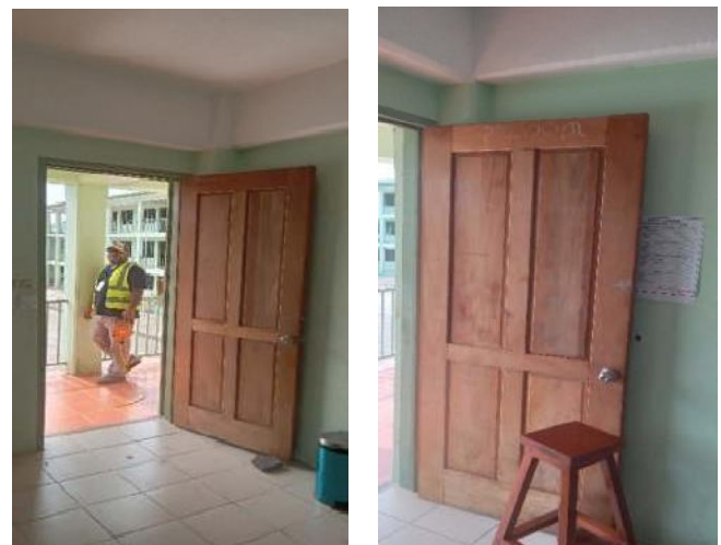
06. SOLID CORE ACCESS DOORS HUNG ON SSS HINGES.
