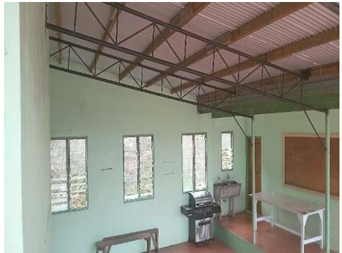
04. ROOF FRAMING OVER WASH BAY.
