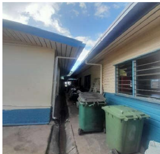
04. BLOCK 03 &amp; LIBRARY STORM DISCHARGE INTO DRAIN.
