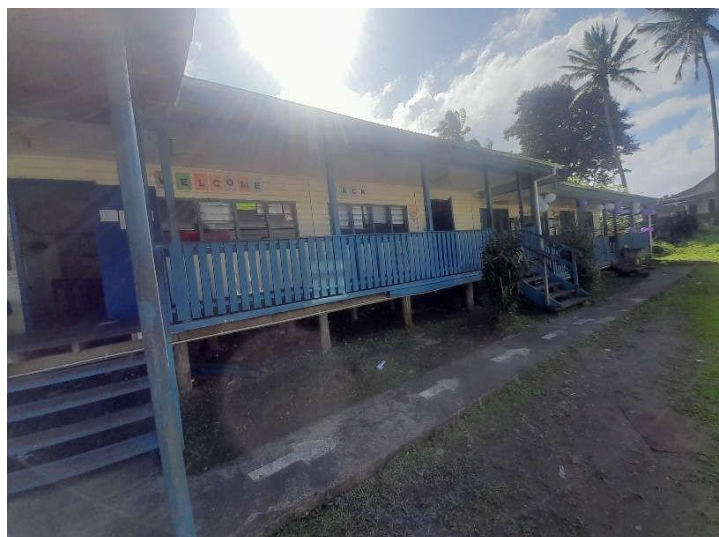
03. TIMBER FLOOR RAISED ABOVE GROUND.
