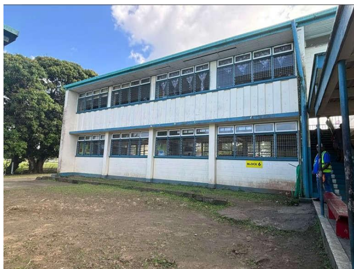
01. WINDOWS ALONG SIDE WALLS, MISSING DOWN PIPES.
