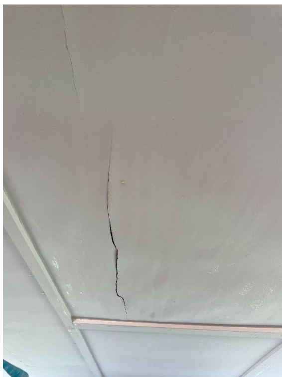
PHOTOGRAPH No. 9: DEFECTS Shown here is a visible hole on ceiling possibly due to leakages
