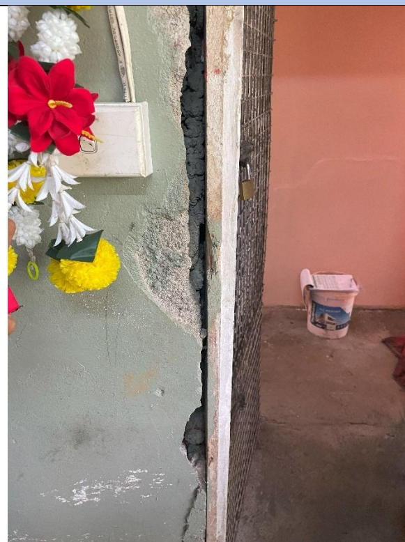
PHOTOGRAPH No. 10: DEFECTS Shown here is a damaged concrete along door frame
