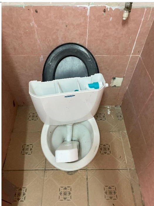
PHOTOGRAPH No. 9: DEFECTS Shown here is a damaged cistern
