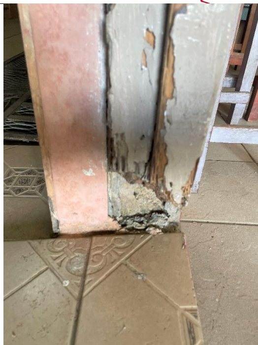
PHOTOGRAPH No. 10: DEFECTS Shown here is a deteriorated timber door frame
