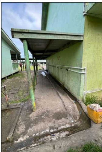
03. TAPS ON SIDE WALL & WATER TANK SUPPLY.
