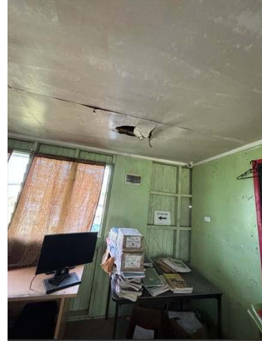
06. DAMAGED CEILING DUE TO ROOF LEAK.
