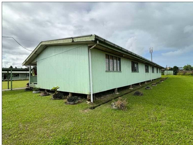
02. BACK VIEW, FLOOR RAISED ABOVE GL.
