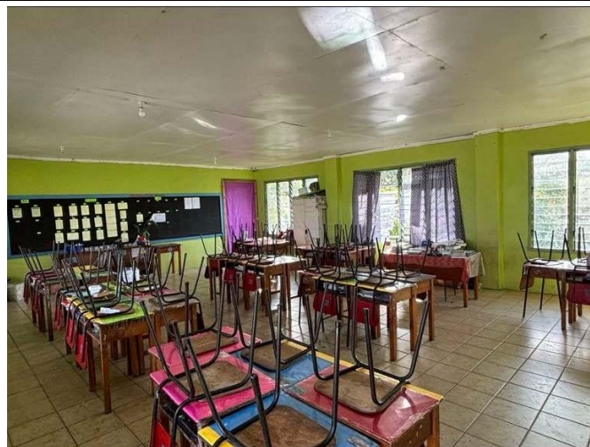
04. YEAR 602 - TILED FLOOR, CEILING U/S ROOF FRAME.
