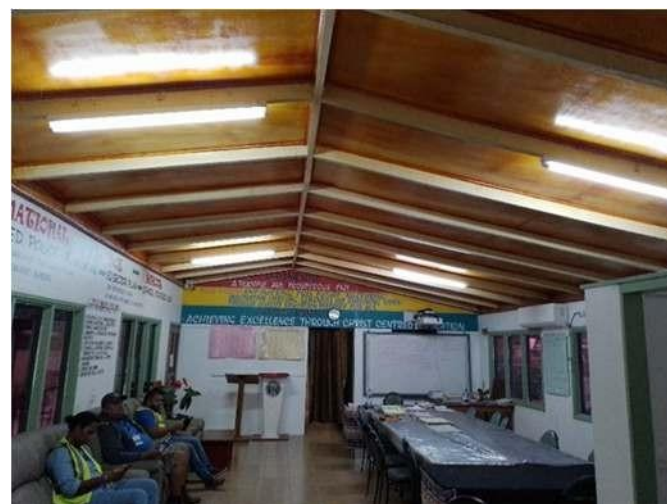
05. EXPOSED CEILING FOR MOST PART OF ADMIN BLOCK.
