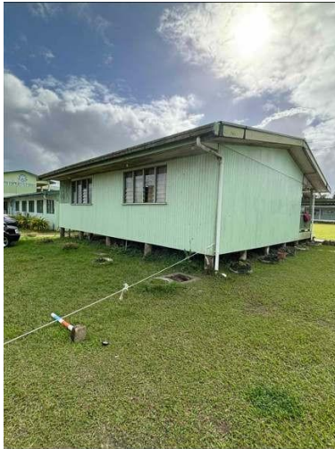
03. BACK VIEW, FLOOR RAISED ABOVE GL.
