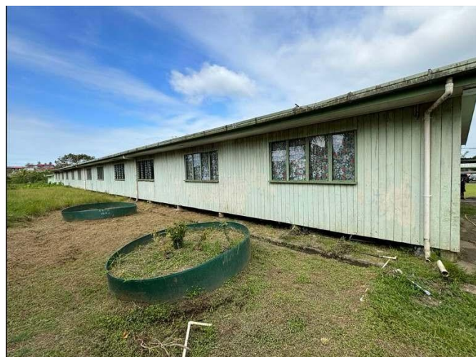
02. BACK VIEW, FLOOR RAISED ABOVE GL.
