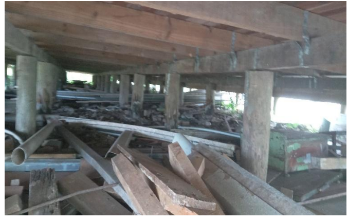
04. TIMBER SUB FLOOR FRAMING & TIE DOWNS.
