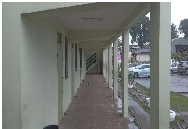
03. RIGID CONCRETE BEAMS & COLUMNS STRUCTURE.
