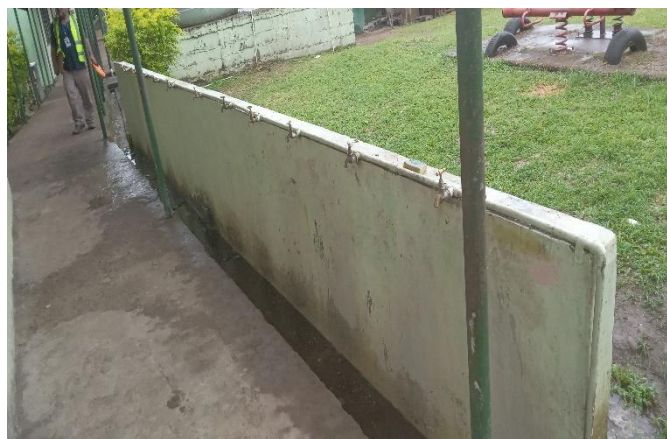
02. BACKUP SUPPLY TO HAND WASH POINT.
