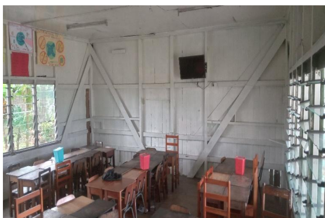
05. END & SIDE WALL TIMBER FRAME.
