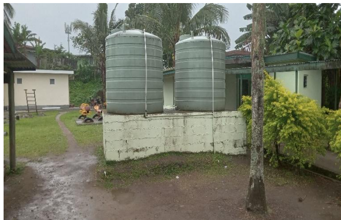
02. BACKUP SUPPLY TO HAND WASH POINT.
