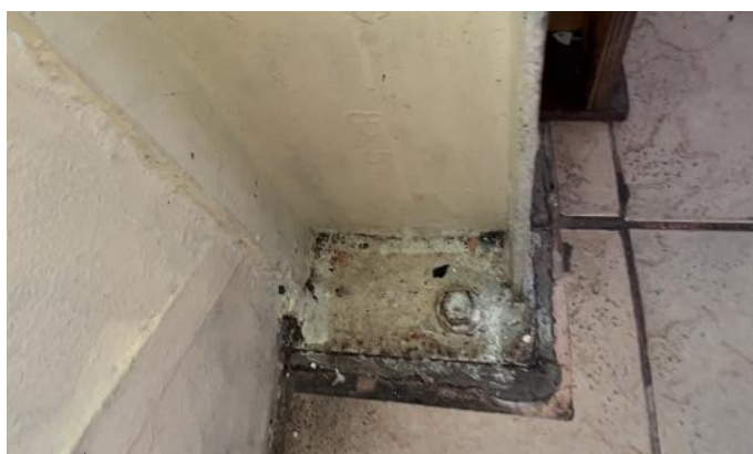
Figure 7: B1 COLUMN BASE PLATE CONNECTION.
