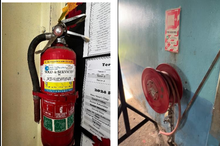
Figure 17: B1 FIRE EXTINGUISHER AND FIRE HOSE REEL.
