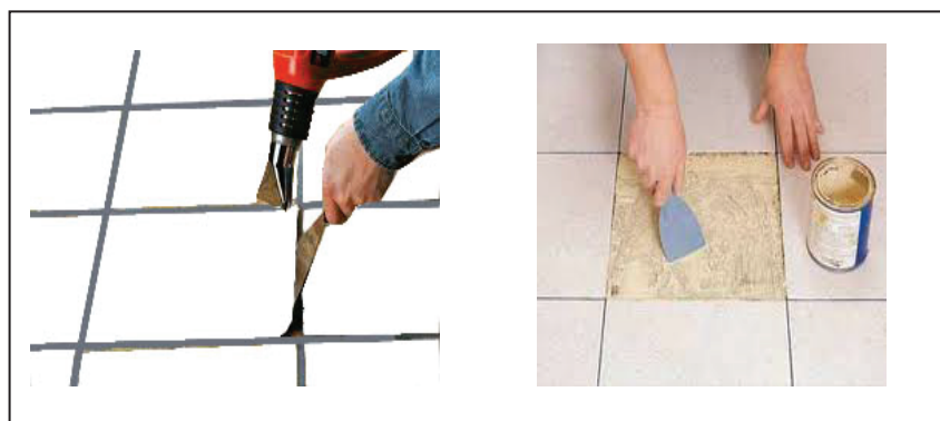
Picture 27: Replacing vinyl tile.
