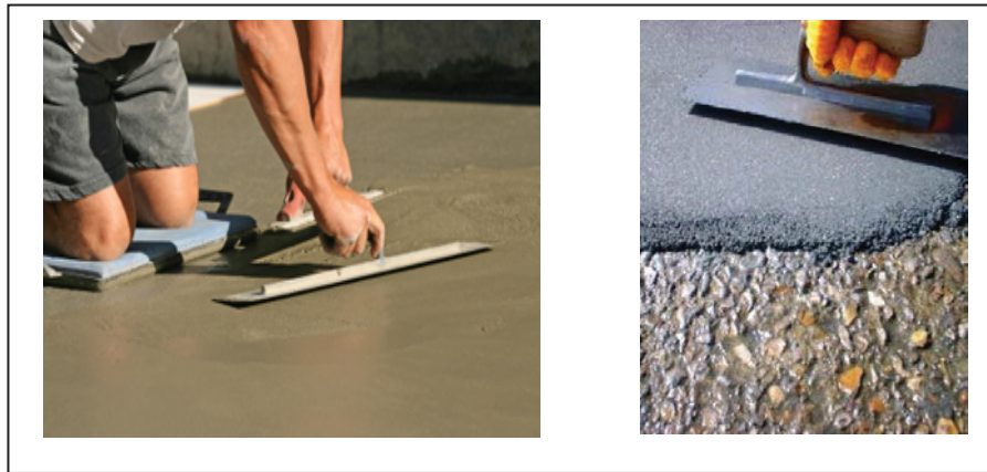
Picture 28: Resurfacing the concrete floor.
