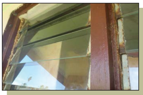
Picture 22: Corroded louvers frame.
