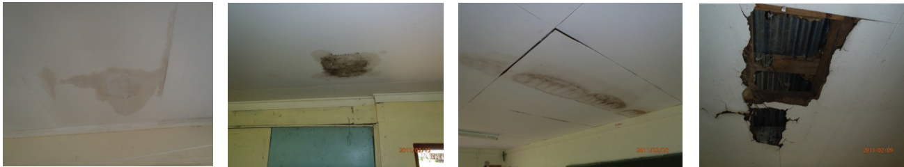
Picture 6: Leaking roof and marks on the ceiling.
