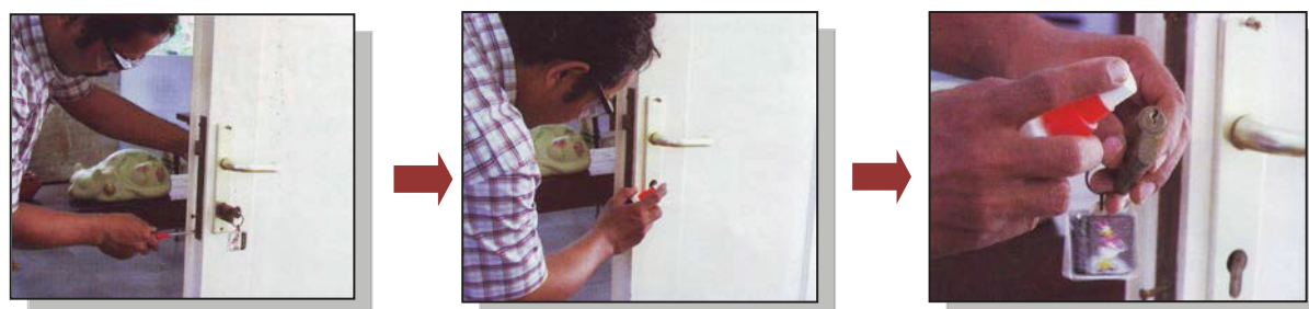
Picture 19: Fixing a mortise lock.
