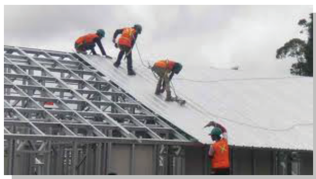
Picture 10: Changing the roof sheets.
