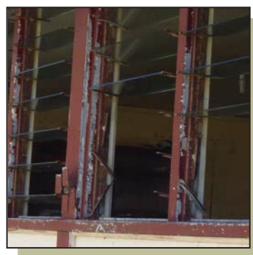
Picture 23: Damaged louver holders.
