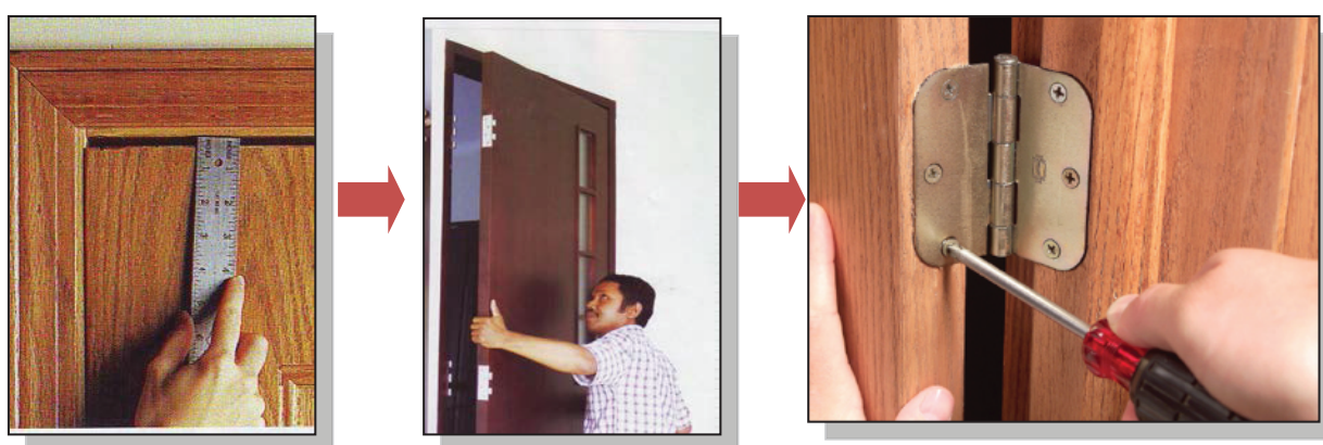
Picture 20: Fixing the door hinges.
