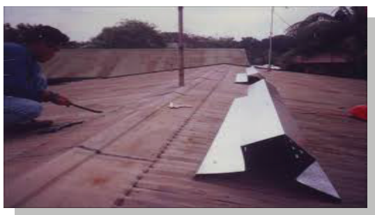
Picture 9: Removing roof nails.
