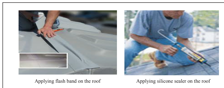
Picture 7: Application of flash bands and Silicon sealer on the roof.
